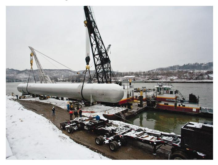
area to the dock location. Using stout cables rated at more than 300 tons, each tank was lifted onto a separate barge. I-beam saddles were then welded to the tanks and freight ships to prevent any movement onboard while the cargoes were under way. Then it was off to Steubenville, a thousand waterborne miles upstream, more or less.
